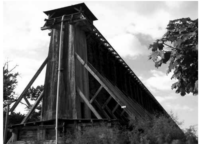
Fig. 2. Cooling Tower in Czechohynek (Poland)
